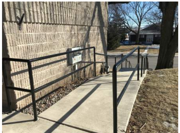
FIGURE 12: Exterior concrete sidewalk/stair/metal railing appear to be in good condition.
