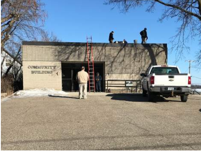
FIGURE 1: Overall exterior view at Community Center entrance.
