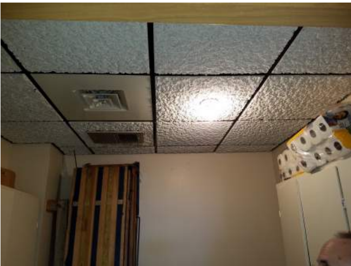
FIGURE 44: Recommend replacement of light with led bulb.
