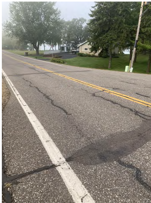
Figure 5: CSAH 7 Existing Road Condition
