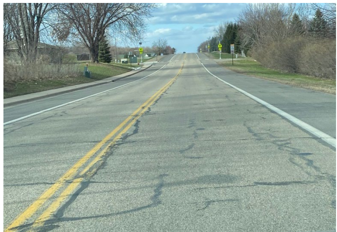
Mill & Overlay completed 2018
