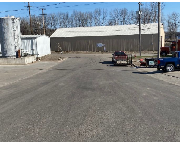
Pavement Reconstruction completed 2019
