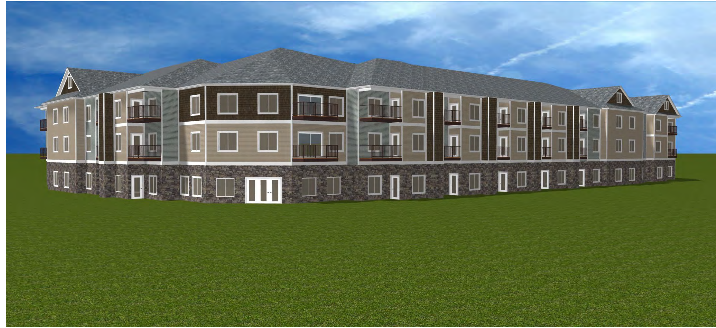
REAR SIDE OF BUILDING 'A'
