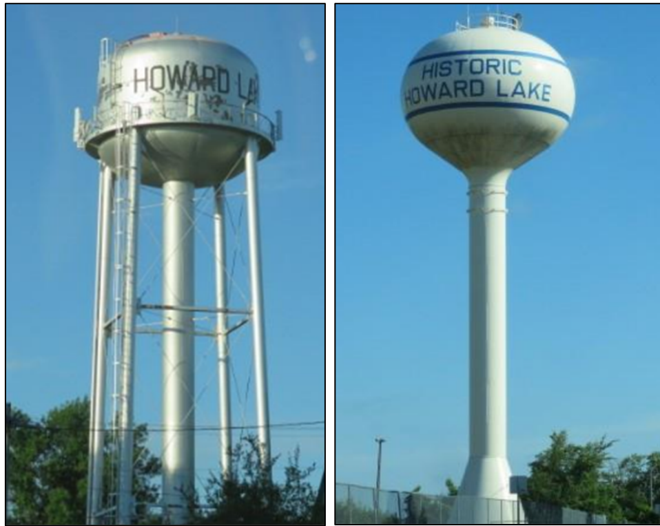
Figure 3.3 Photo of tower No. 1 on the left.
